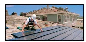
Roof integrated photovoltaics replacing roof material
