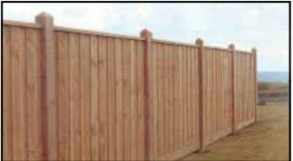
Timber paling fence with exposed posts
