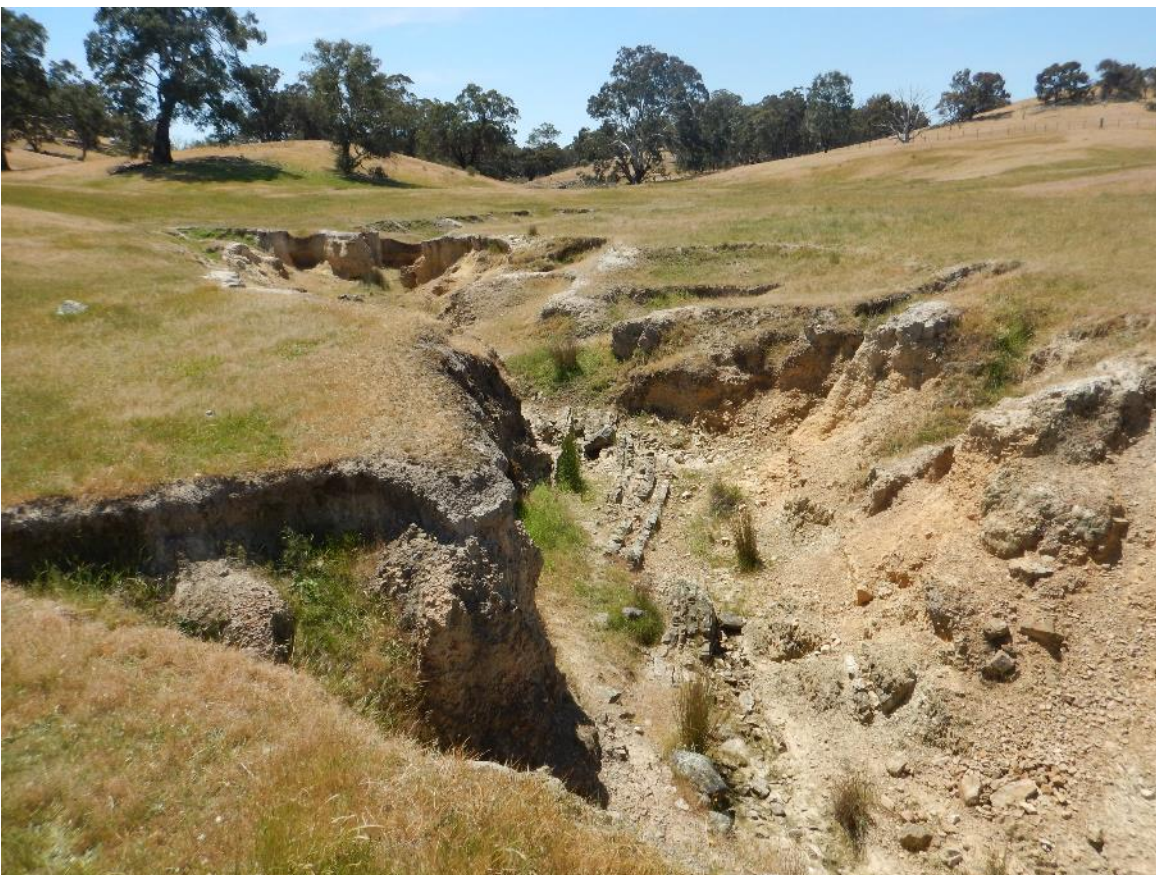
Photo 12 Collapsed tunnels excluded from the central portion of the offset area.
