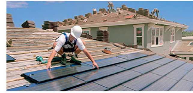
Roof integrated photovoltaics replacing roof material
