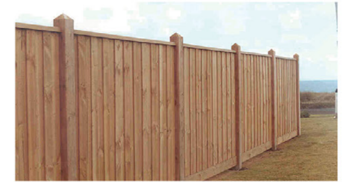
Timber paling fence with exposed posts
