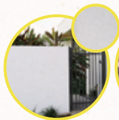
LOT WALLS Rendered masonry walls, painted white
