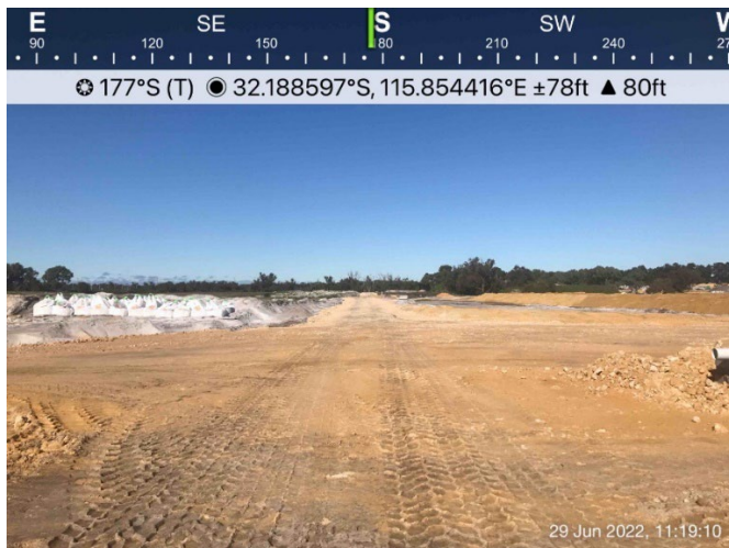
Plate 2: EAW connection with Magnificent Drive in the north (facing south)
