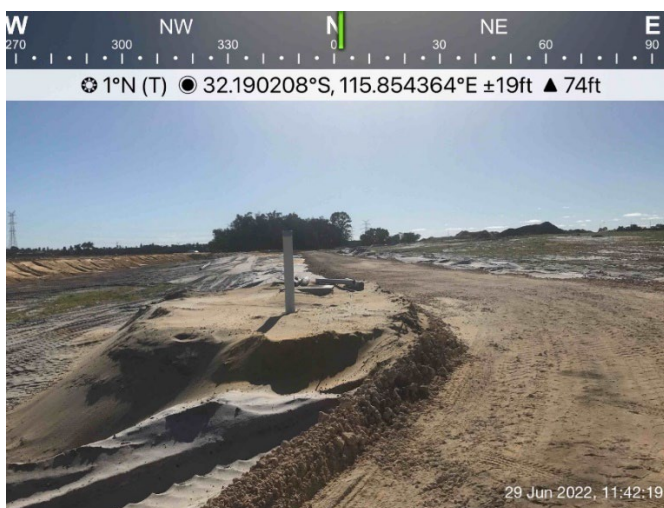
Plate 3: Central section of EAW (facing north)
